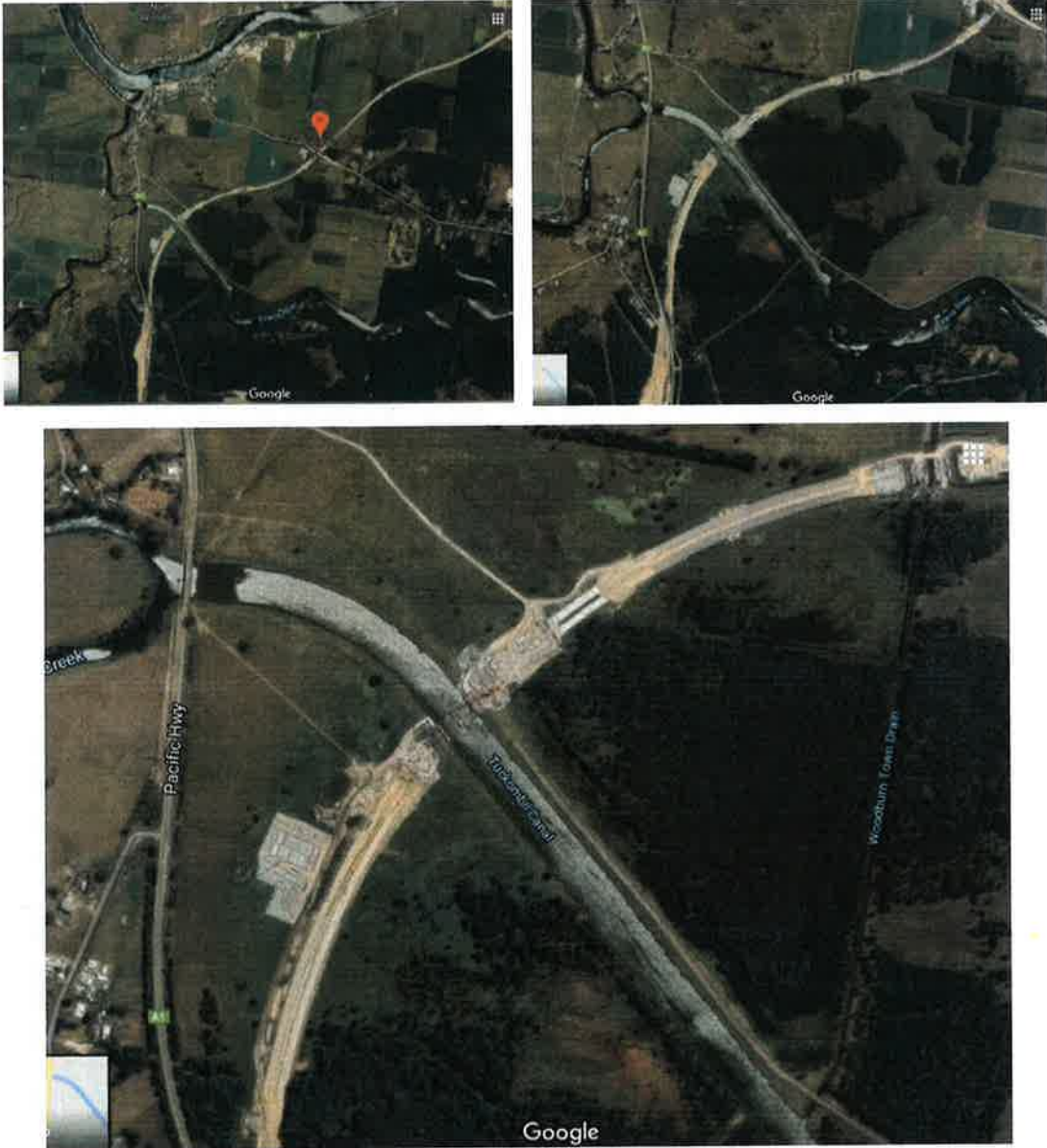
Fig 7. Highway over the Canal showing three escapes, the canal bridge, a small escape to its north and the bridge over the Woodburn Town Drain
