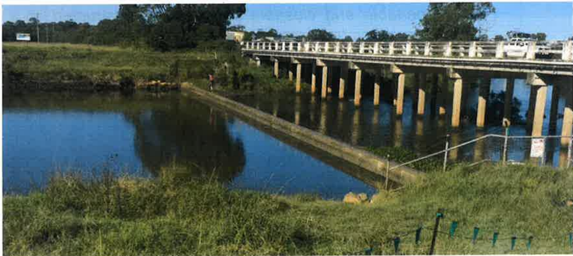
Fig 16 Tuckombil Canal Fixed Concrete Block Weir
