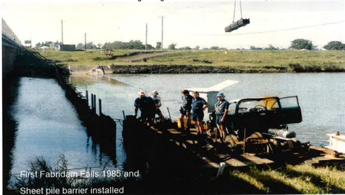
Fig 5 Steel Sheet Pile Barrier – 1985 (Michael Woods Photo)
